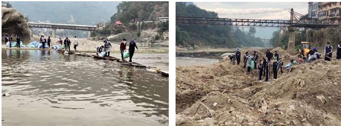
Reduced manpower successfully resulting cleanup operation.
